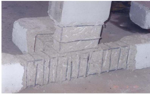
(a) Removing the concrete cover for beams and column
