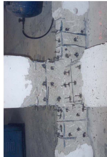
(a) Removing the concrete cover for beams and column
